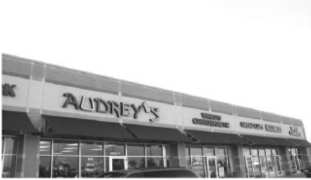
Discouraged: Flat roof and no significant fascia or cornice
