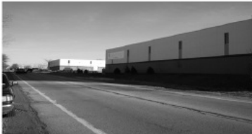
Discouraged: Long, blank building walls visible from adjacent major roadway
