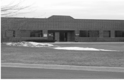
Discouraged: Parapet conveys a two-dimensional appearance
