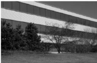
Discouraged: Inadequate building setback and landscaping
