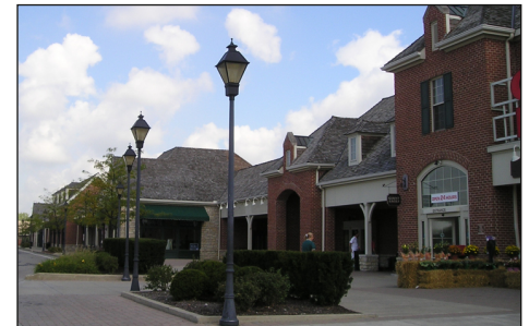
Pedestrian-scaled architecture in both urban (above) and suburban (below) settings.
