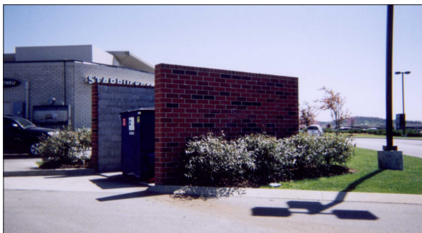
Figure 14 & 15: Screened Refuse Area
