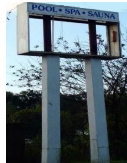
Example of Abandoned Sign
