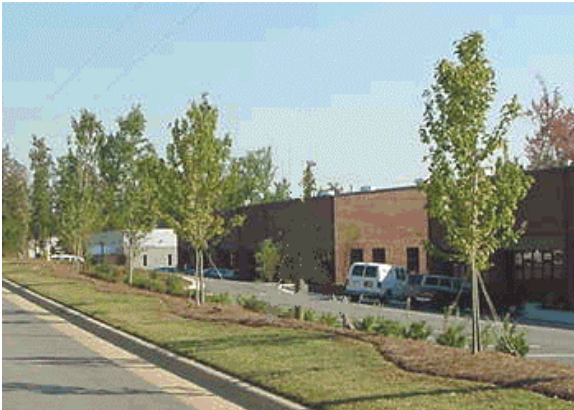
Example of Type 1 – Open Landscaping
