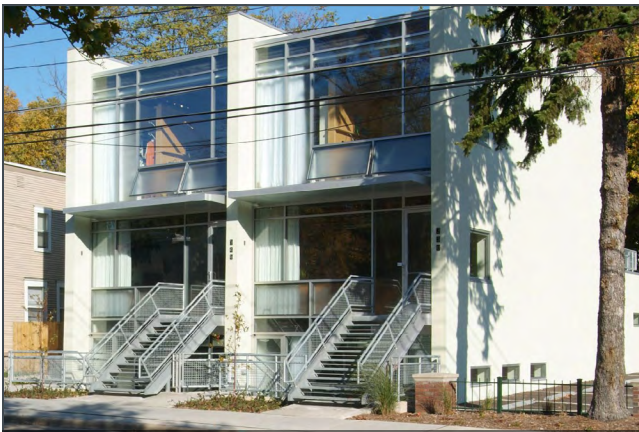
ROWHOUSE BUILDINGS WITH LIGHTWELL FACADES
