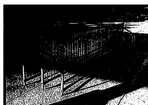
Bike racks, like those shown to the left, are not easy to use, do not adequately support bicycle frames or protect bicycles from damage. Use of these types of bicycle racks shall be avoided.
