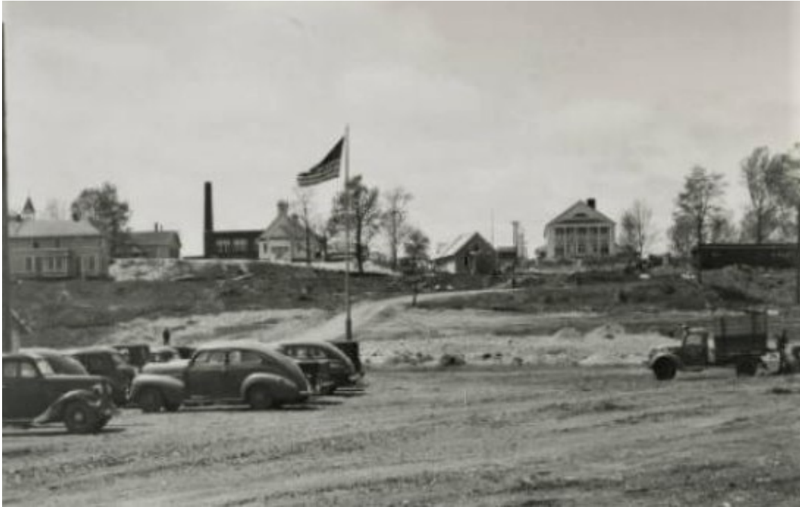
Construction of the Ford Plant in Big Bay, MI
