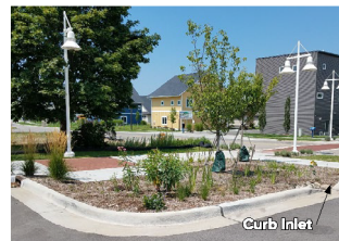
Source: Macatawa Area Coordinating Council Parking Lot Island Rain Garden, 16th Street
