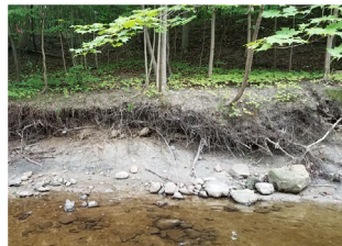
Tulip Intercountry Drain, Holland, MI Source: Macatawa Area Coordinating Council (MAAC)
