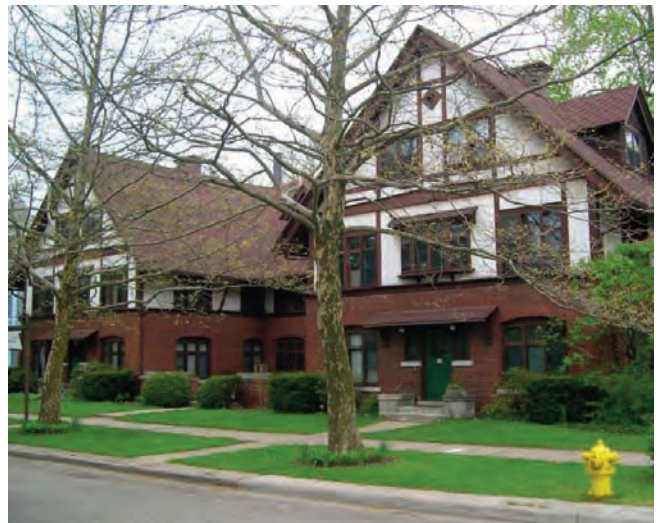
IMAGE 6.144 APARTMENT BUILDING TYPE
