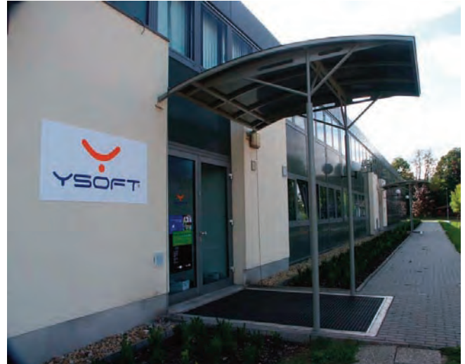
IMAGE 6.231 INDUSTRIAL SHOP TYPE CANOPY
