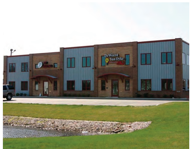
IMAGE 6.216 INDUSTRIAL SHOP BUILDING TYPE
