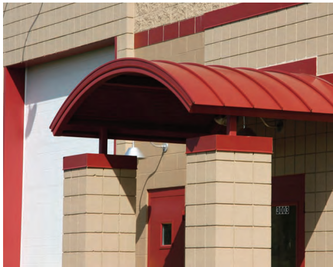
IMAGE 6.234 INDUSTRIAL SHOP TYPE ENTRY
