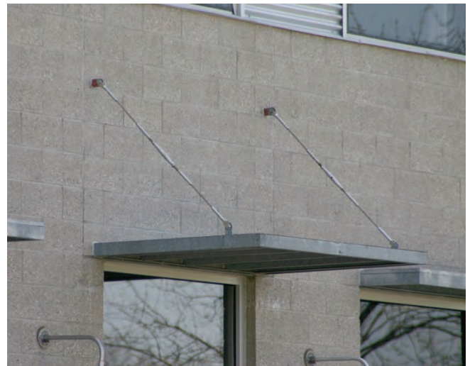
IMAGE 6.233 INDUSTRIAL SHOP TYPE CANOPY
