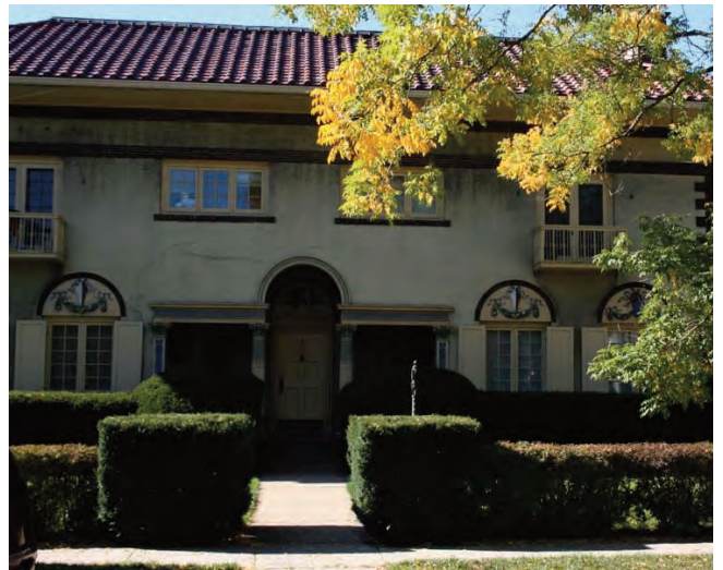
IMAGE 6.143 APARTMENT BUILDING TYPE
