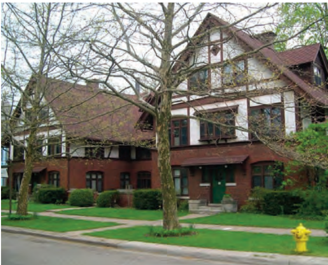
IMAGE 6.134 APARTMENT BUILDING TYPE
