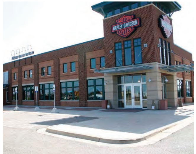
IMAGE 6.224 INDUSTRIAL SHOP BUILDING TYPE
