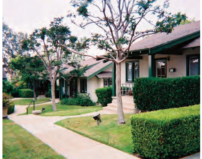
IMAGE 6.197 COTTAGE HOUSE TYPE STOOP
