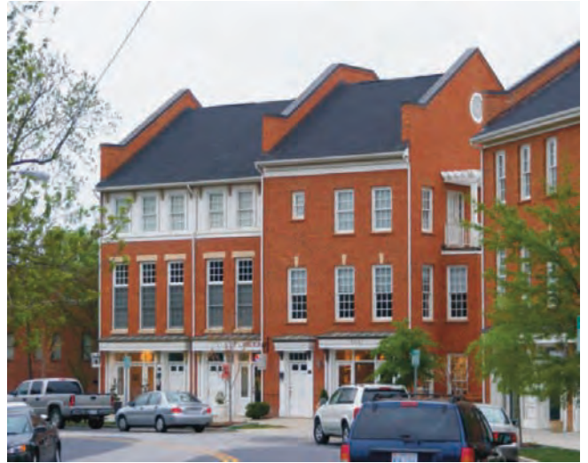
IMAGE 6.112 LIVE-WORK TYPE FRONT FAÇADE
