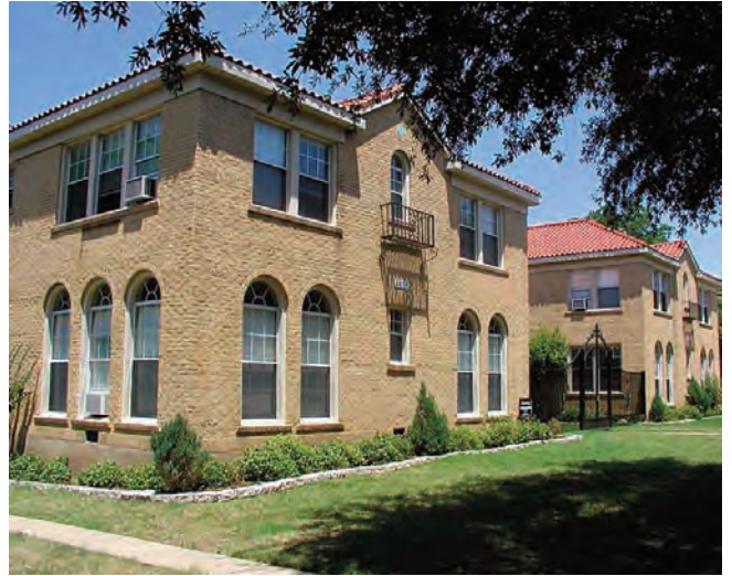
IMAGE 6.142 APARTMENT BUILDING TYPE
