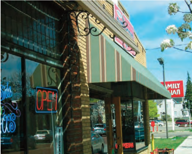
IMAGE 6.35 MIXED USE BUILDING TYPE AWNING
