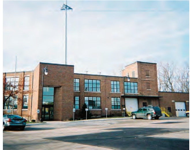
IMAGE 6.214 INDUSTRIAL SHOP BUILDING TYPE
