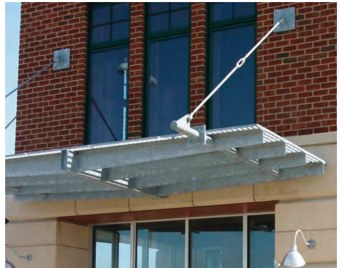
IMAGE 6.232 INDUSTRIAL SHOP TYPE CANOPY
