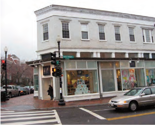
IMAGE 6.14 MIXED USE BUILDING TYPE MASONRY
