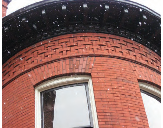
IMAGE 6.177 ROWHOUSE TYPE CORNICE
