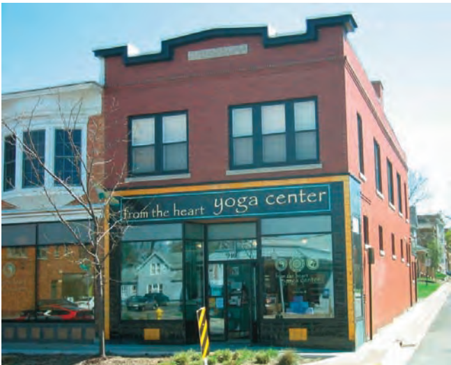
IMAGE 6.15 MIXED USE BUILDING TYPE MASONRY
