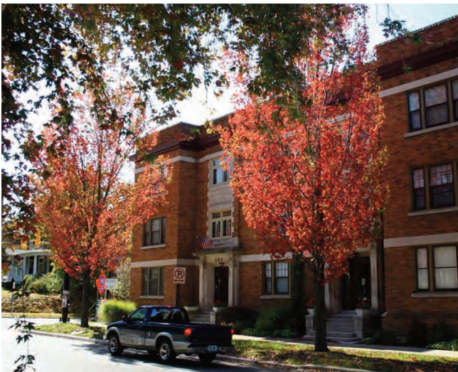
IMAGE 6.141 APARTMENT BUILDING TYPE
