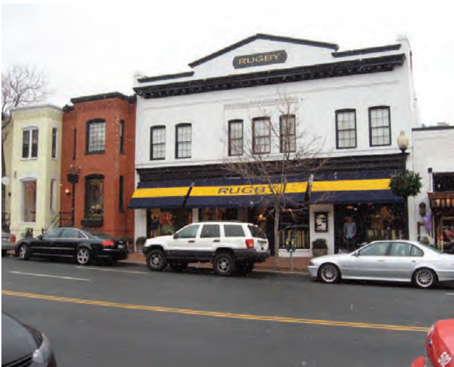
IMAGE 6.16 MIXED USE BUILDING TYPE MASONRY
