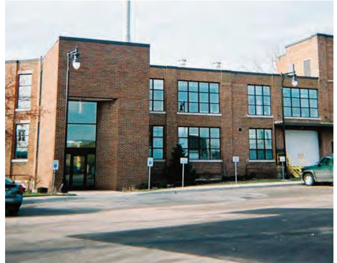
IMAGE 6.222 INDUSTRIAL SHOP BUILDING TYPE
