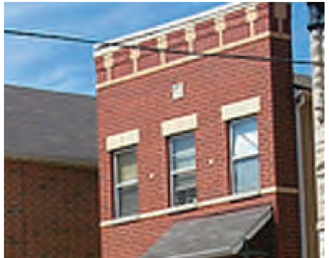
IMAGE 6.178 ROWHOUSE TYPE CORNICE
