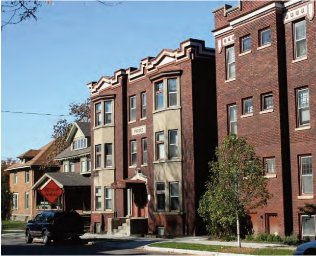
IMAGE 6.139 APARTMENT BUILDING TYPE
