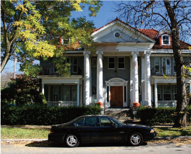
IMAGE 6.132 APARTMENT BUILDING TYPE
