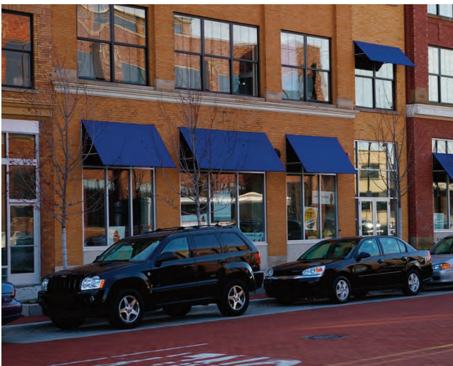
IMAGE 6.36 MIXED USE BUILDING TYPE AWNING
