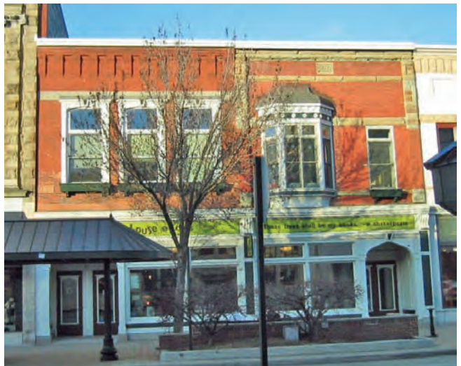
IMAGE 6.19 MIXED USE BUILDING TYPE MASONRY
