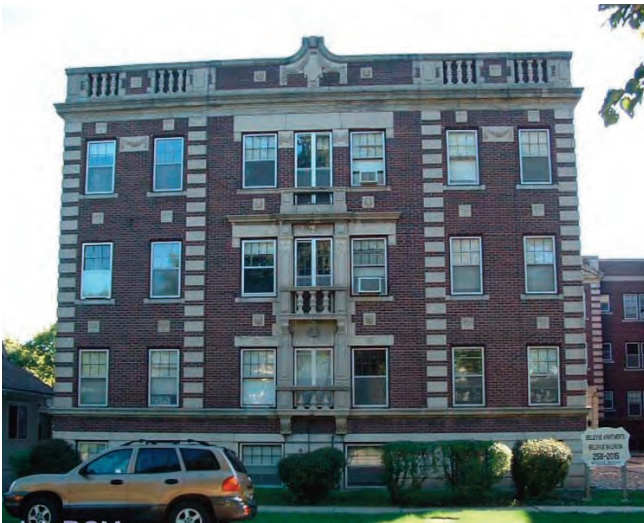
IMAGE 6.140 APARTMENT BUILDING TYPE
