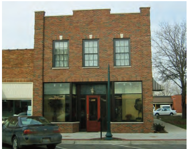
IMAGE 6.18 MIXED USE BUILDING TYPE MASONRY
