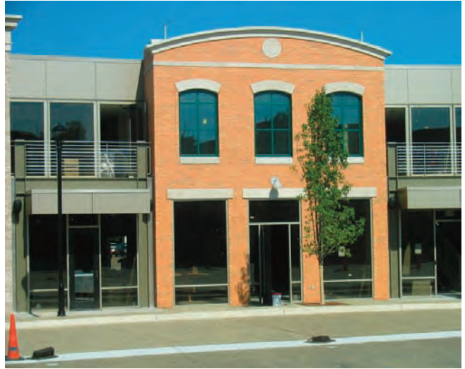
IMAGE 6.17 MIXED USE BUILDING TYPE MASONRY
