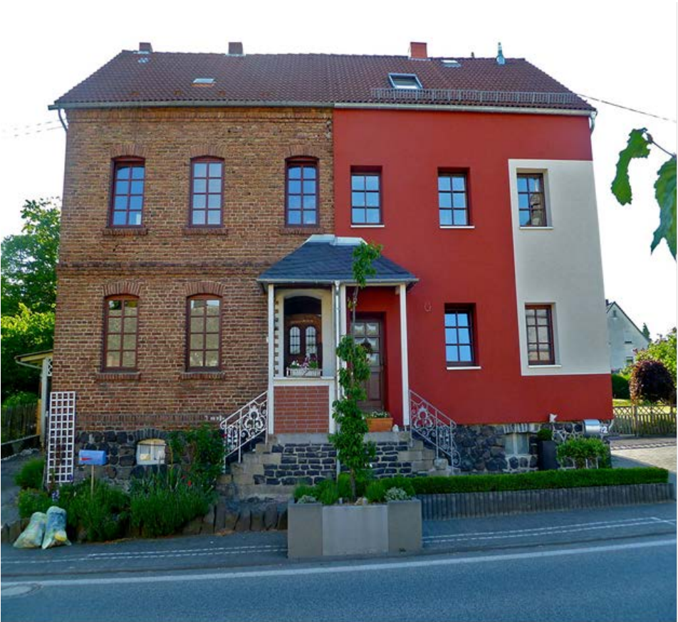
EFIS on right side. (Exterior Finish and Insulation Systems)
