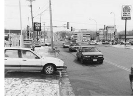
Figure 15.8 Image from a Minnesota Department of Transportation document explaining the benefits of Corridor Access Management shows the consequences of poor planning decisions along a commercial thoroughfare including uncoordinated development, traffic conflicts, erratic design standards, inconsistent signage, and the absence of landscaping.
