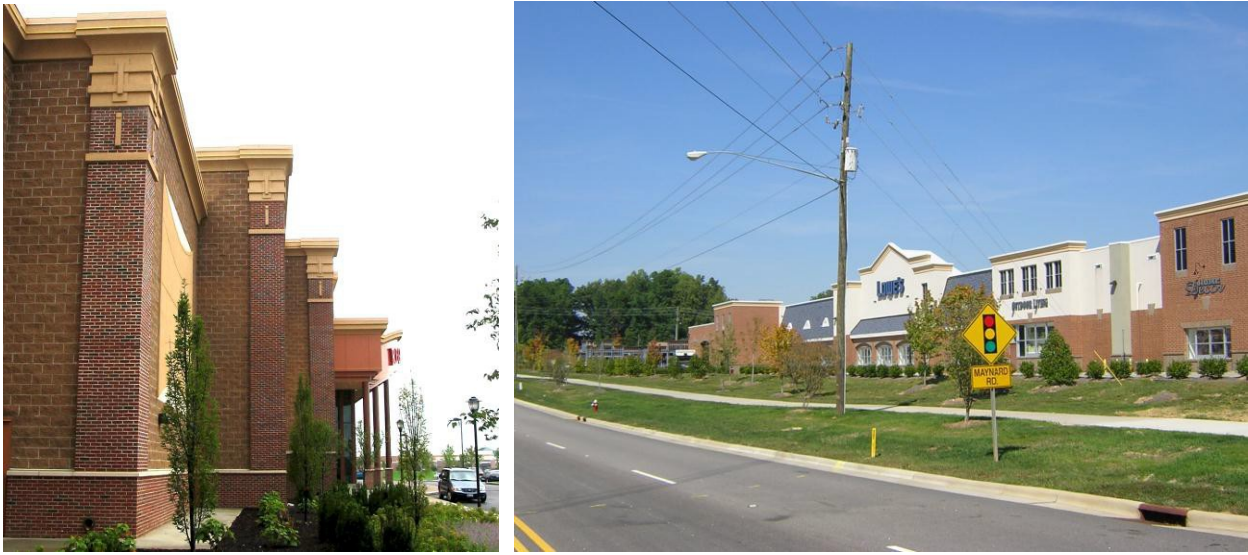
Figure 9-1: The buildings in the above images contain pilasters, cornices, and a series of façade setbacks (recesses) to visually break up the appearance of large facades.
