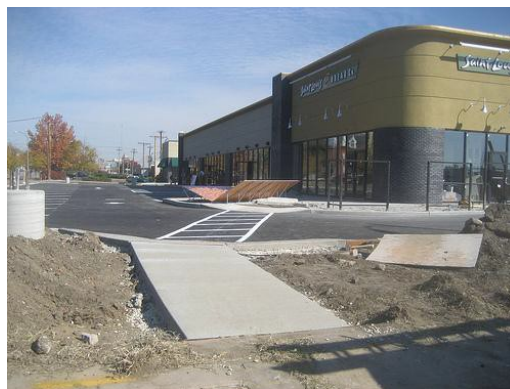
Figure 11-2: This image illustrates a sidewalk connection between a building and a public sidewalk in the right-of-way. This connection includes both a separate sidewalk (foreground) and a connection delineated through a painted line (background).
