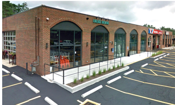
Figure 3B: Example of Building After Modifications
