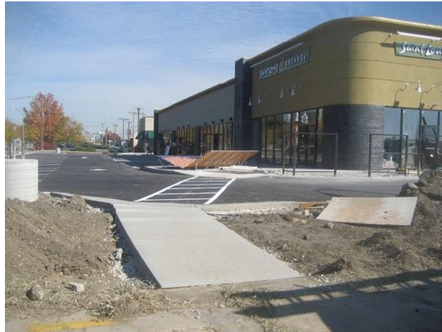
Figure 9.04-3: This image illustrates a sidewalk connection between a building and a public sidewalk in the right-of-way. This connection includes both a separate sidewalk (foreground) and a connection delineated through a painted line (background).
