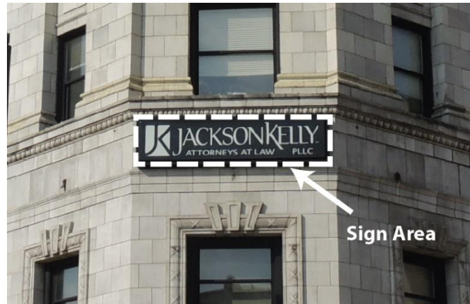
Figure 1304-B: Illustration of computing sign area for wall signs with a background panel or cabinet.
