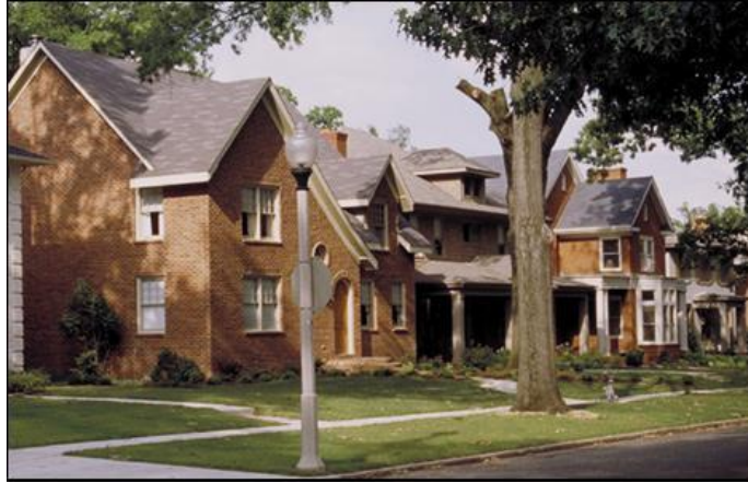
Figure 906-A: The detached dwelling in the foreground exhibits compatibility with the surrounding dwellings in regard to design, scale, setbacks, and materials.
