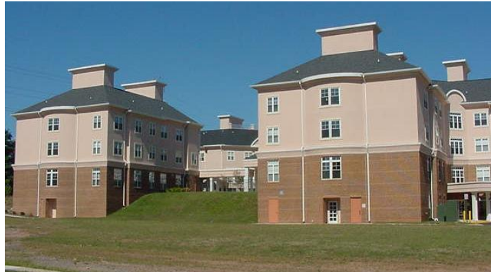
Figure 6.05-2: This multi-family development lacks sufficient façade variation yielding a monotonous appearance
