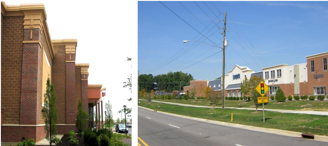
Figure 10.04-1: The buildings in the above images contain pilasters, cornices, and a series of façade setbacks (recesses) to visually break up the appearance of large facades.
