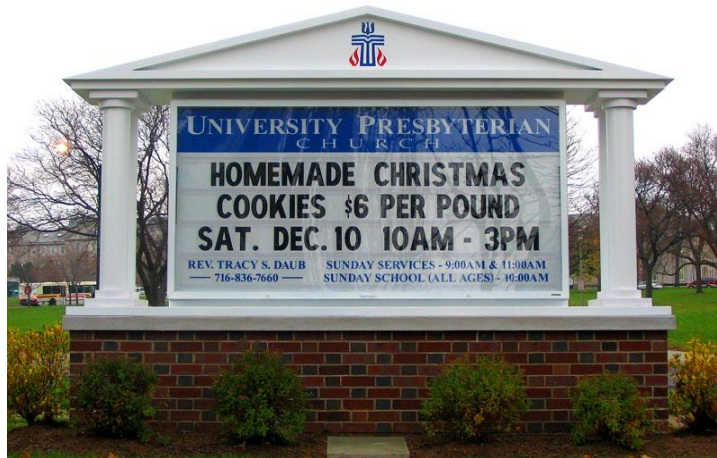
Figure 13.07-1: Illustration of a sign for an institutional use on a brick base with foundation plantings.
