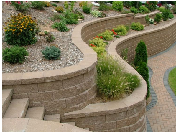
Figure 9.05-1: Retaining shall be benched, or terraced, so that no individual wall exceeds a height of six feet.
