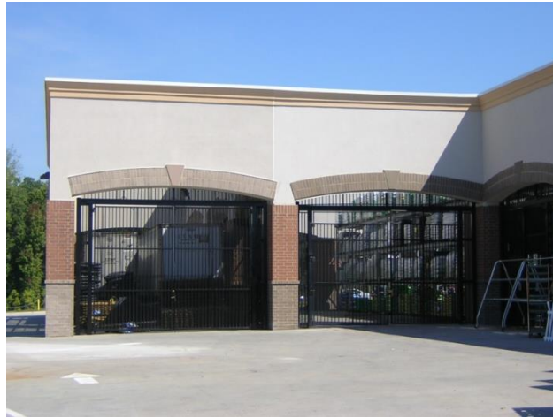
Figure 12.08-1: Use of a wall and fencing for screening that is architecturally compatible with the principal building.
