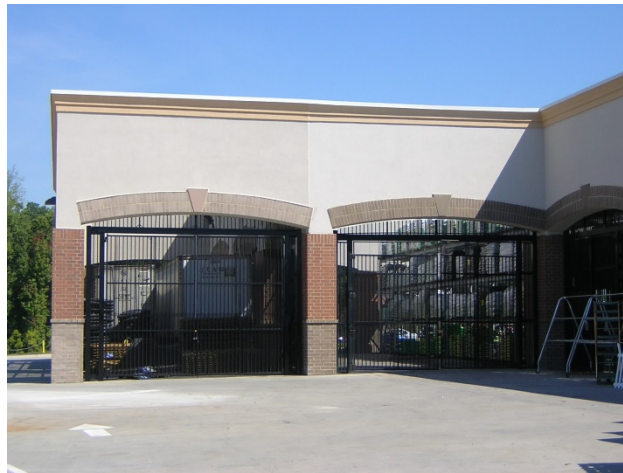
Figure 8.06-A: Use of a wall and fencing for screening that is architecturally compatible with the principal building.
