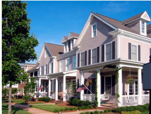
Figure 4.08-C: This image illustrates how multiple design features are incorporated to de-emphasize the fact that this is a single structure.
