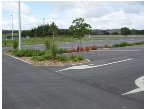
Figure 12.02-C: Example of a rain garden incorporation with parking lot landscaping.
