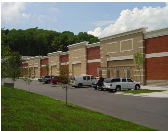
Figure 6-16: This figure shows two methods of using architectural features to create wall surface relief on wall elevations that are not the primary elevation.
