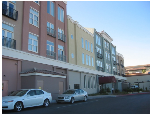
Figure 6-16: This figure shows two methods of using architectural features to create wall surface relief on wall elevations that are not the primary elevation.
