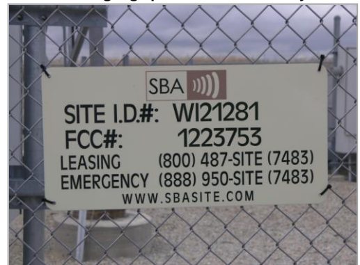
Exhibit 7-9. An example of appropriate tower signage placed on the security fence
