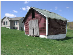
Exhibit 5-1. An example of a rural accessory building
