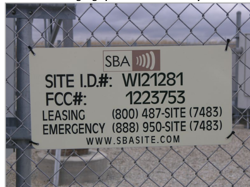
Exhibit 8-7. An example of appropriate tower signage placed on the security fence
