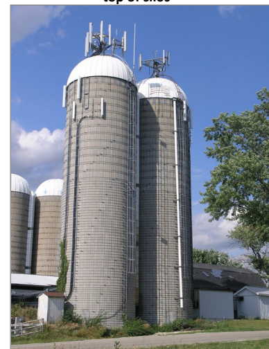
Exhibit 3-2. Two antenna arrays on top of silos
